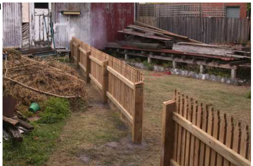
Some of the demolition materials (the fence was to keep our dog away from blackberries, cars, etc.)
