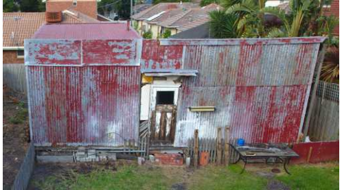
The existing workshed
